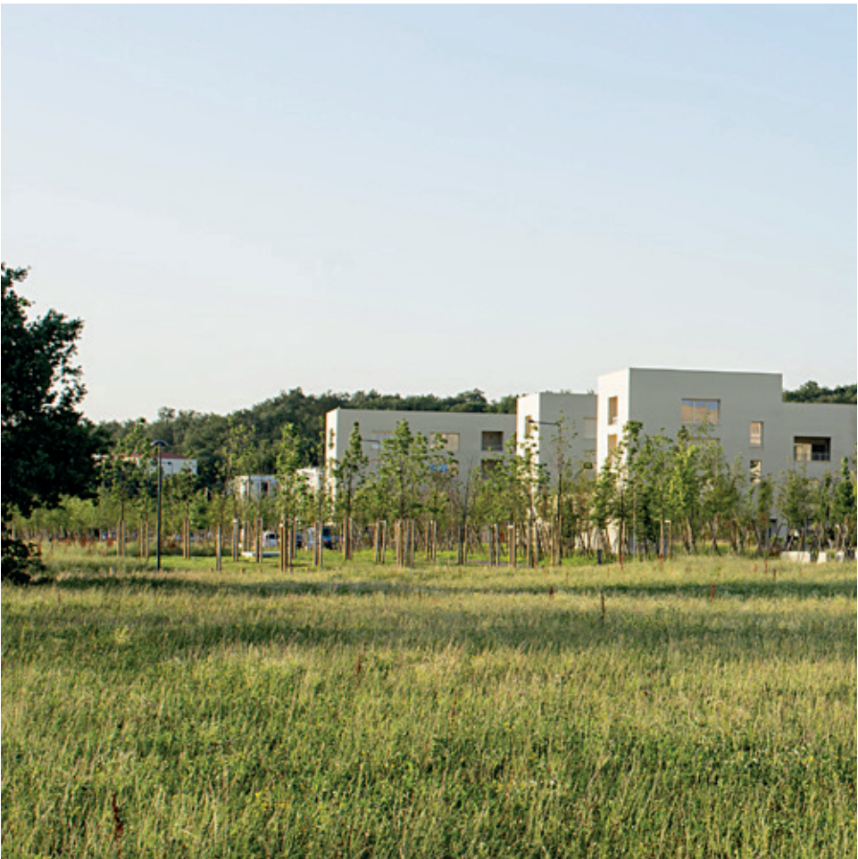
Raphael Gabrion Architectes, Cornebarrieu, France
